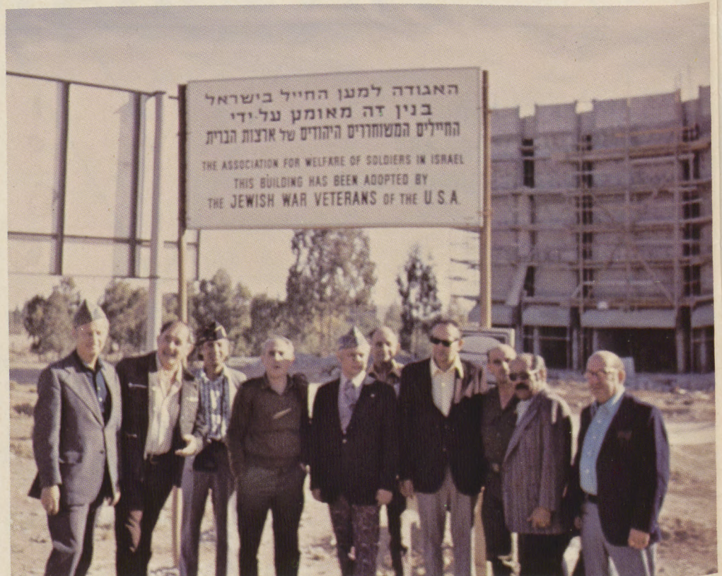
National Commander and party inspect construction of new Beersheba Soldiers Rest Home with Gen. Peri.
